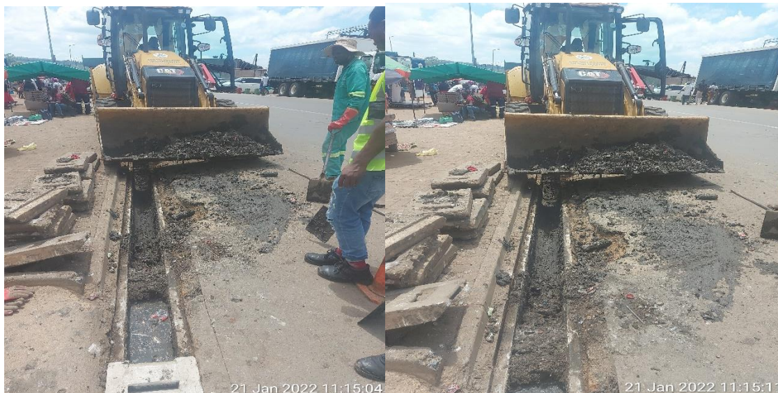
Clearing of storm water drains
